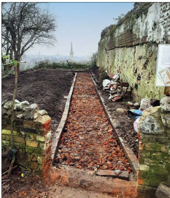
4. A new path was excavated and laid with bricks found around the site
