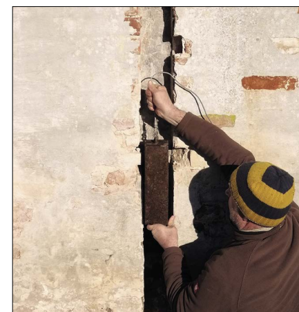
Fig 2. Simon showing the square sash weights in situ.
