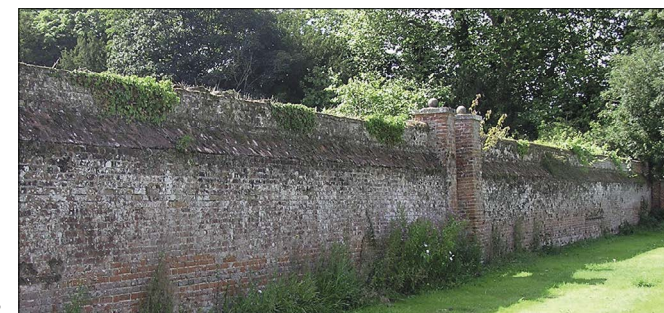
3. The 'hot wall' at Kimberley Hall, inserted into the kitchen garden by Capability Brown in 1778. The fireplaces, evidently for burning coal, given their size, can be seen at the base of the wall in the foreground.
